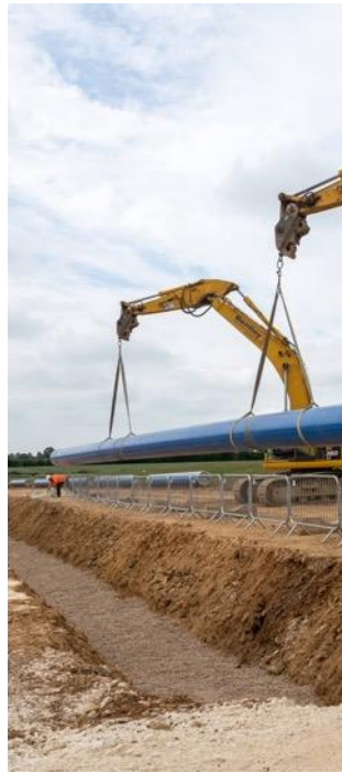
>1,000km of mains renewal
